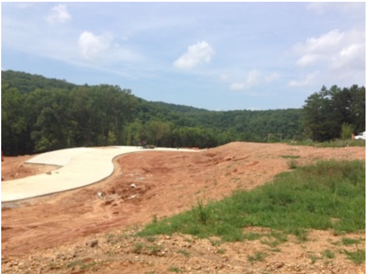
View from the new endpoint of the original walkway, showing the now-terraced slope that will feature the new bioswale.
