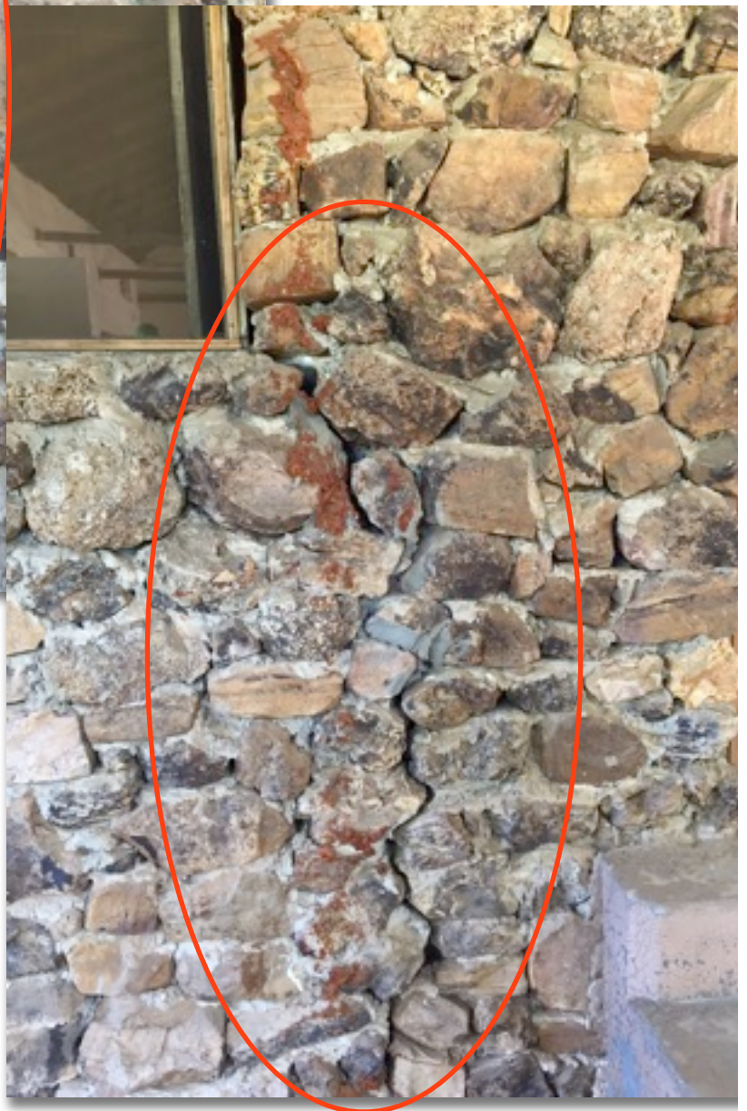
Apparently, at some point there was a misguided attempt to patch it.
